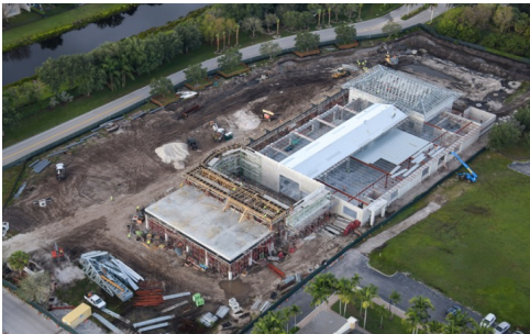
Canyon Branch Library | Boynton Beach, FL | 30k sq. ft | 24M
